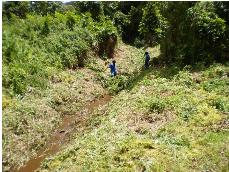
Cleaning of rivulet at Chamarel
